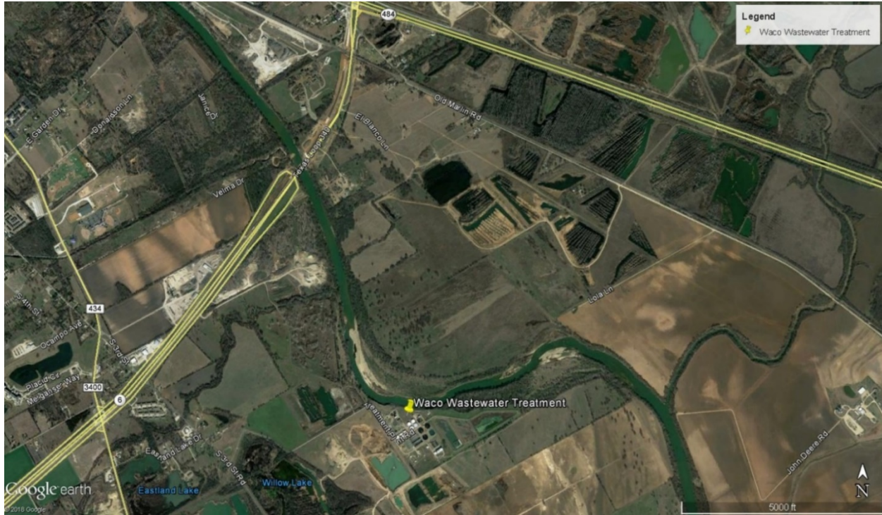
Figure 2. Waco WMARSS Treatment Plant Location
