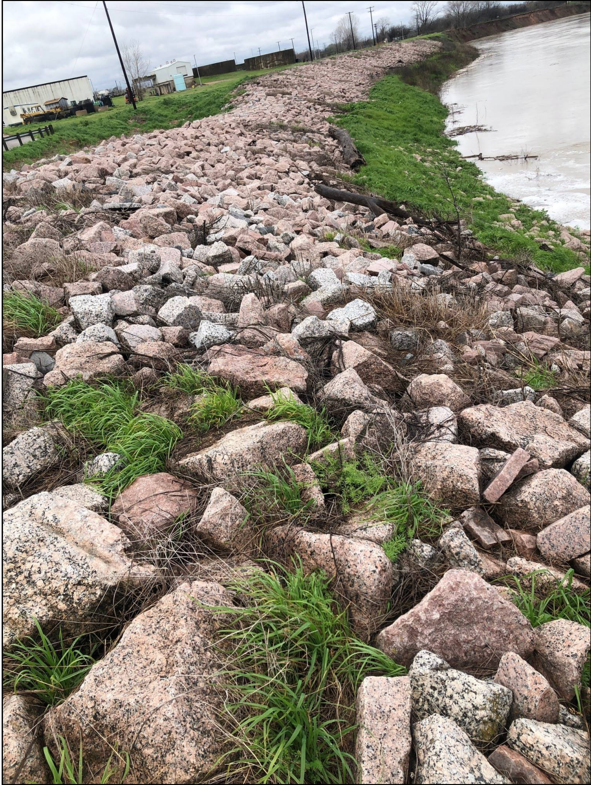
Figure 7. Existing Stream Bank Protection
