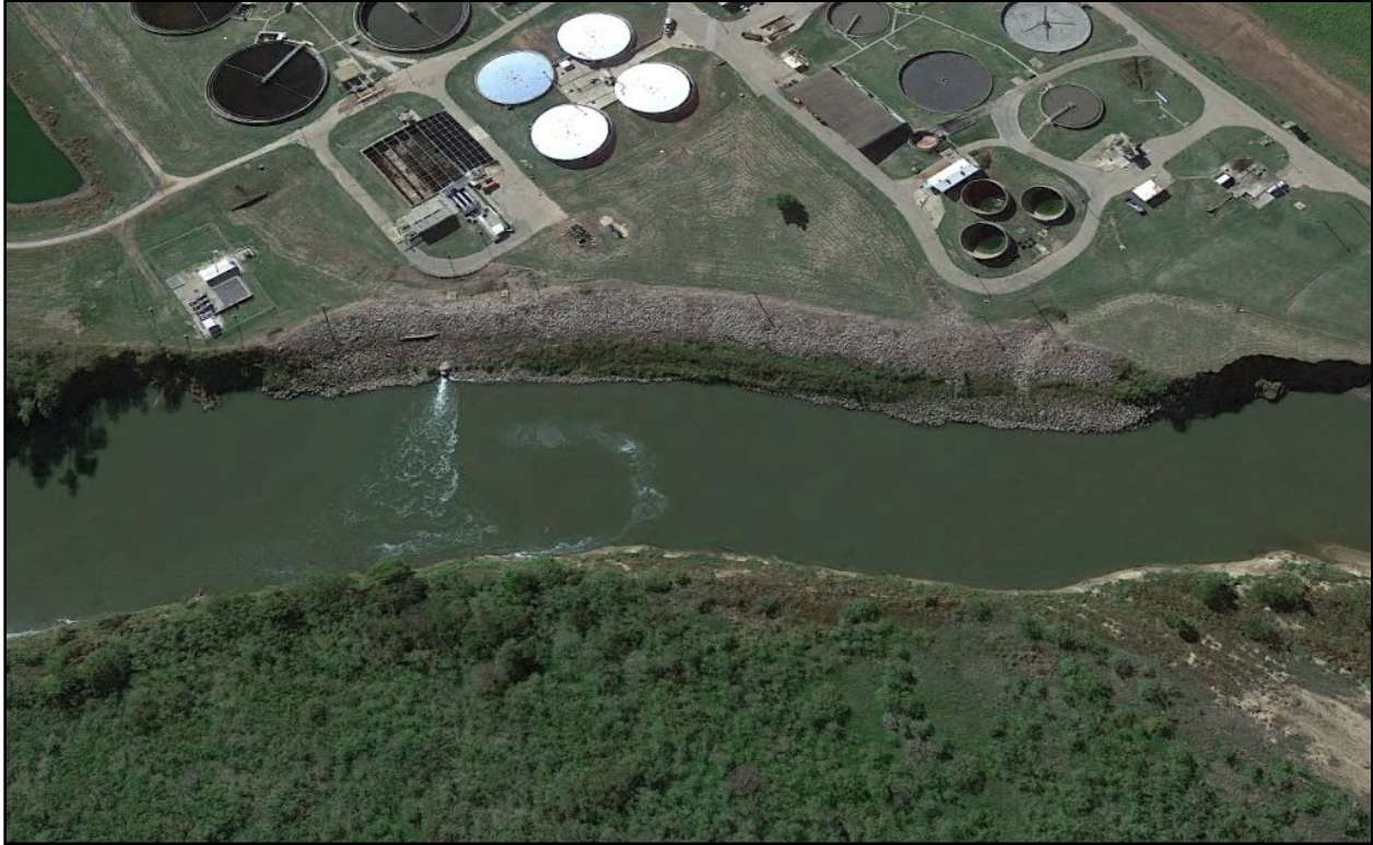
Figure 5. Existing Streambank Protection Project
